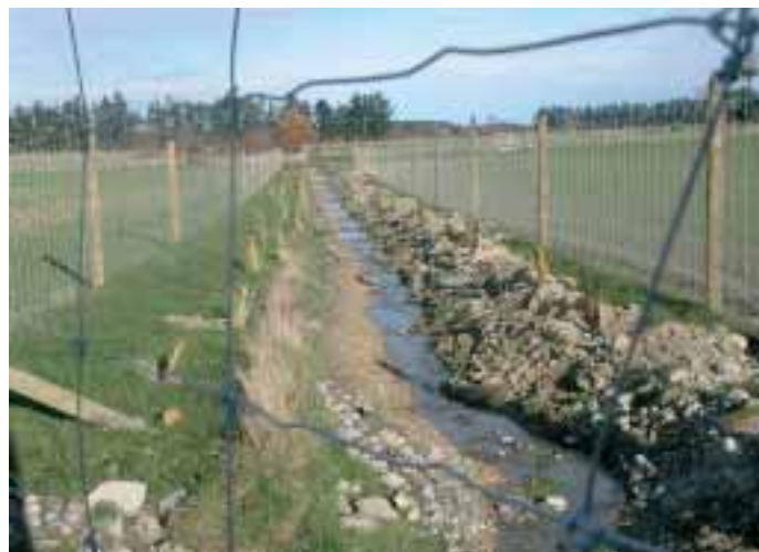
Waterway protection work on Graham Carr's Peel Forest Estate.
