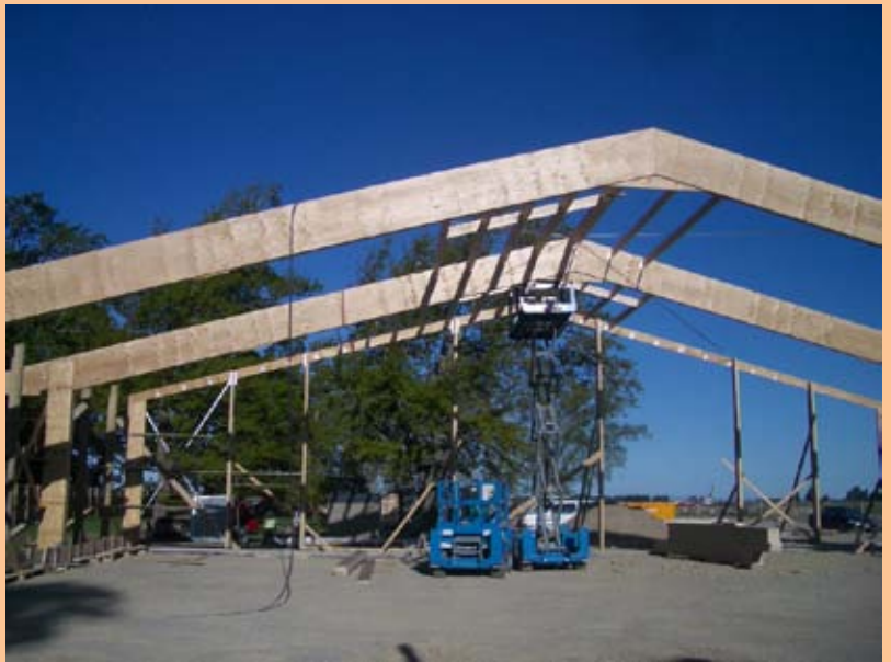
The laminated radiata beams give a 27-metre freespan.
