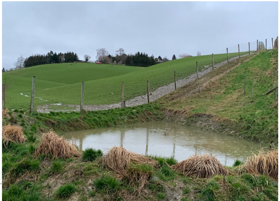
Sediment trap at the bottom of a swale.
