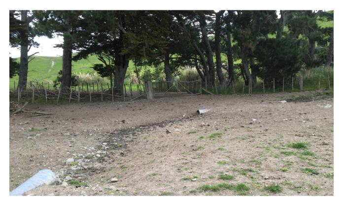
Runoff from a woolshed and sheep yards is captured in this drain and directed into a silt trap. The trap is fenced off from stock and planted (it's visible behind the shelter belt). The silt is periodically scooped out and spread on low-risk paddocks, away from waterways.
