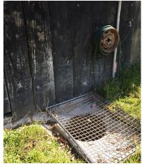
The washdown is then filtered in a sump that can be cleaned out.
