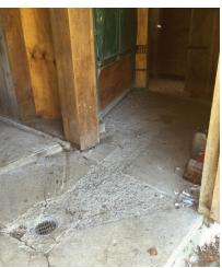
All washdown water from the shed is captured in a drain and directed away from the waterway.
