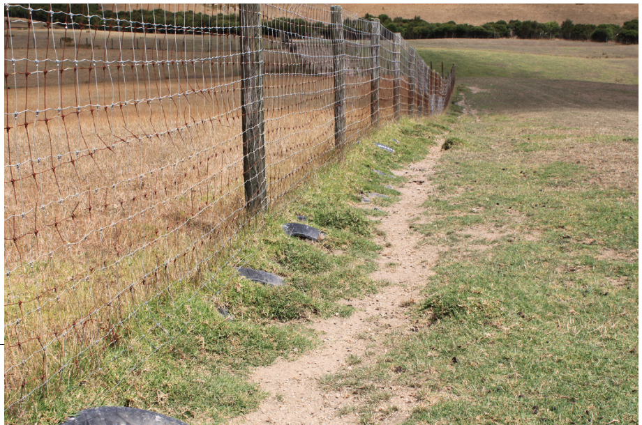
Tyres placed in soil along fence as part of repairs help reduce further pacing.
