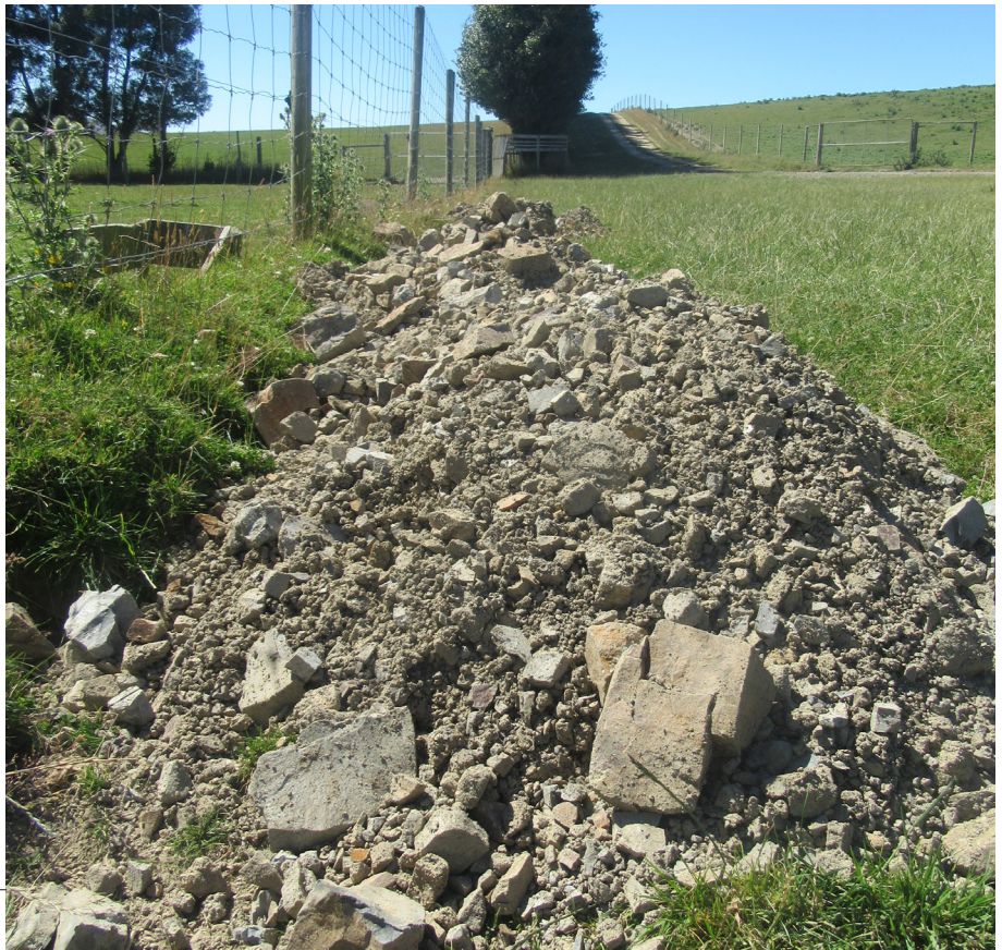
Rock buffer in trench along fenceline.
