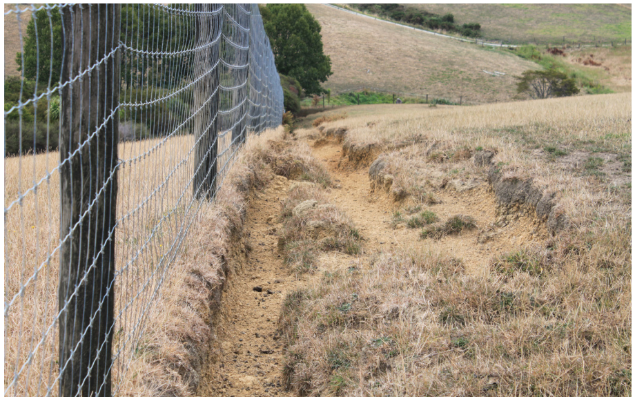
Bad trenching in vulnerable soils caused by fence pacing.
