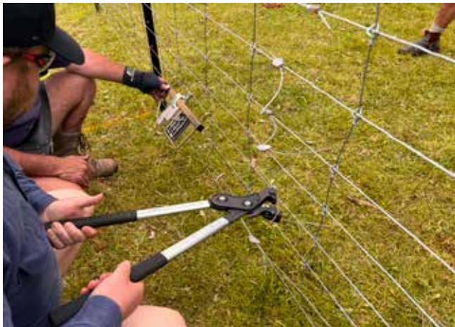
Tie off fencing wire with Bayonet Fastlink Fence Enders.
