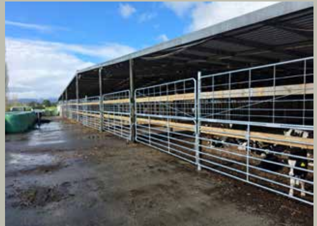
SUPER-SIZED: An exterior view of the 6000 m 2 shed. This year, 900 weaners were wintered in 3000 m 2 . Dairy calves were wintered in 1000 m 2 .
